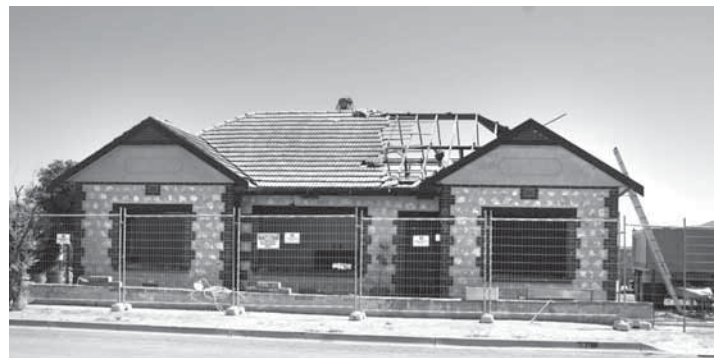
ABOVE: House being demolished
